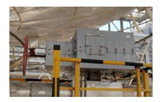
The Daken Epoxy Coating Shell (**DEC**) Passive Fire Protection System is manufactured using a special mouldable, flexible, epoxy intumescent coating system designed to resist the most severe hydrocarbon hazards - pool fires, jet fires and explosions. When exposed to the high temperatures of the fire, the system undergoes a chemical reaction and expands to form a robust, insulating char that reduces the temperature rise of the protected item.
